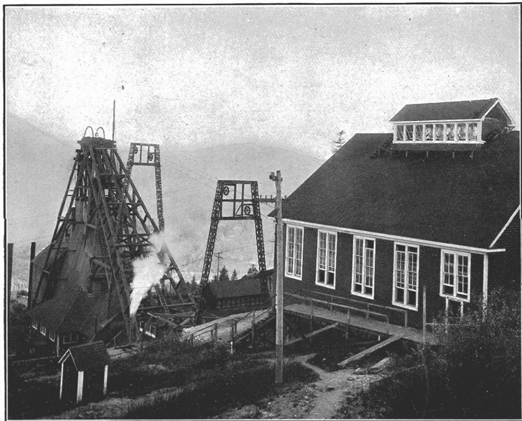
CENTRE STAR HOIST AND HEAD WORKS - ROSSLAND, B.C. Hoist Capacity—1,350 tons from 3,000 feet in ten hours.
