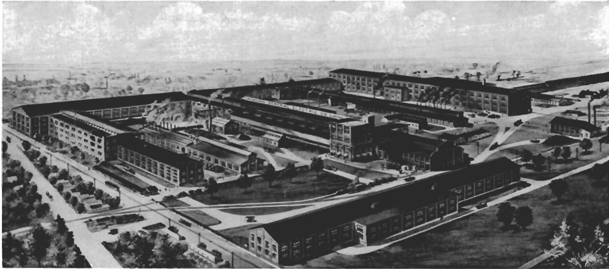
Main Electrical Works, Peterboro, Ont.
