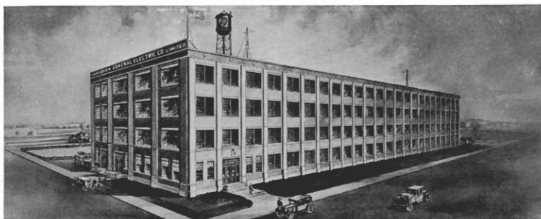
Ward Street Works, Toronto, Ont. Wiring Devices—"Hotpoint" Appliances—"Radiolas"
