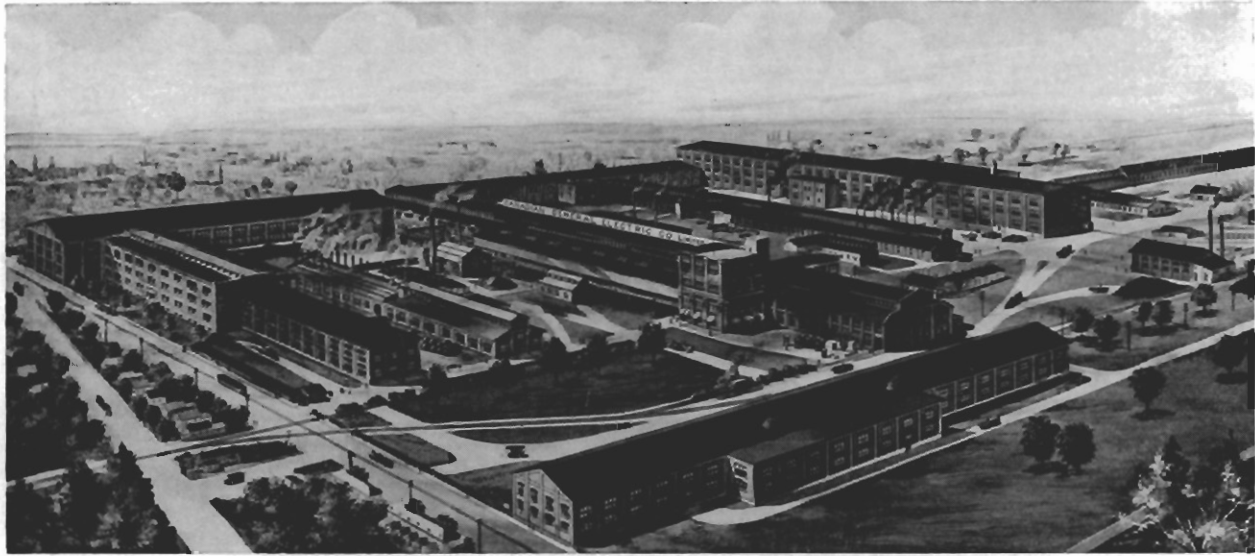
Main Electrical Works, Peterboro, Ont.
