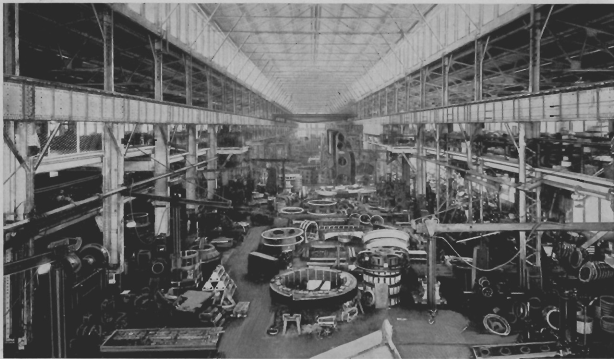
Main Machine Shop—Peterboro Works
