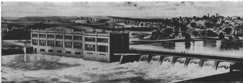
Power House No. 2, Peterboro, Ont.
