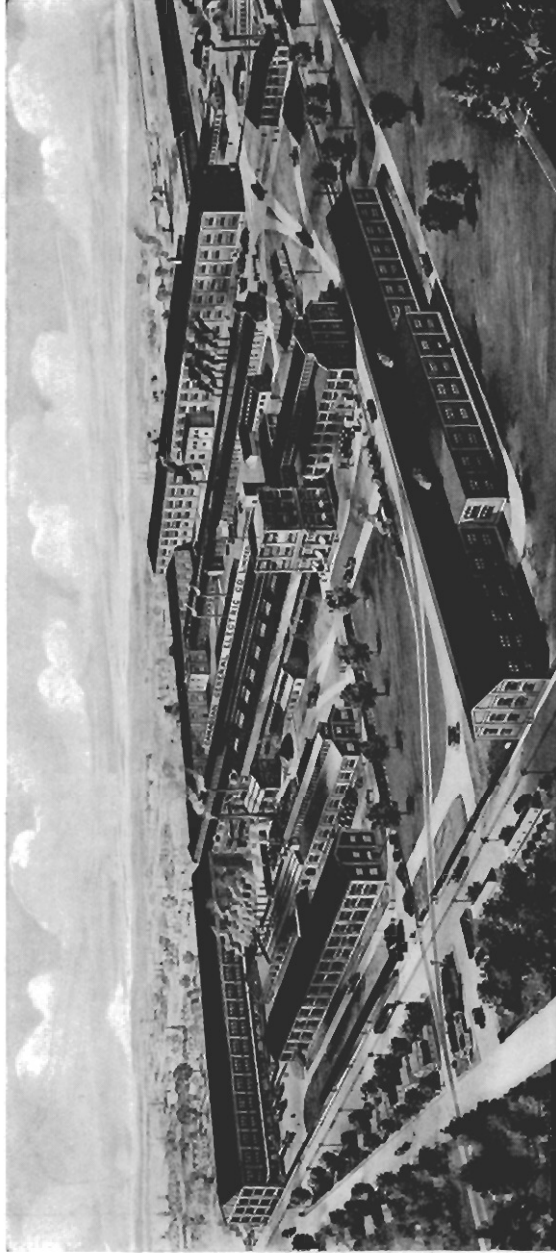
Main Electrical Works, Peterboro, Ont.
