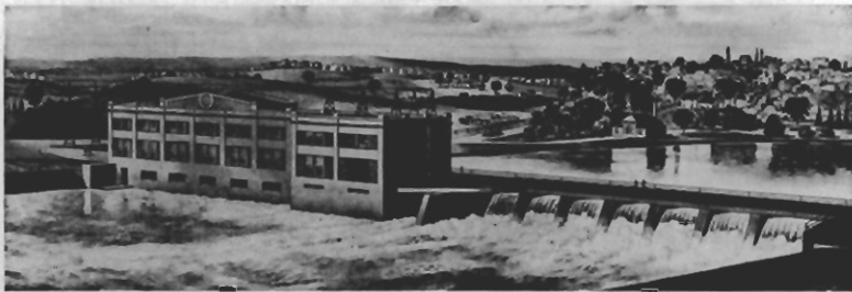
Power House No. 2, Peterboro, Ont.
