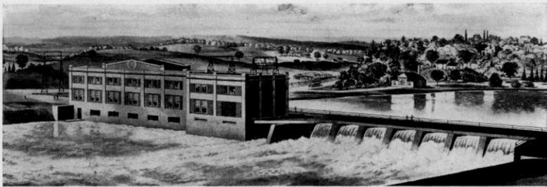
Power House No. 2, Peterboro, Ont.
