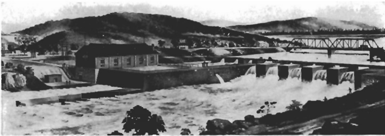
Power House No. 1, Peterboro Ont;
