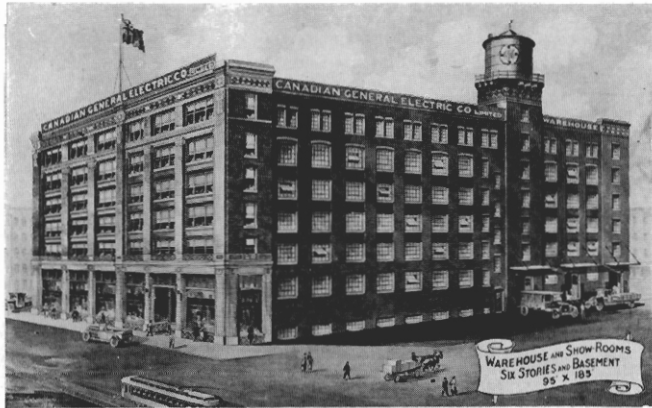
Warehouse and Showroom, 214-218 King St. W., Toronto
