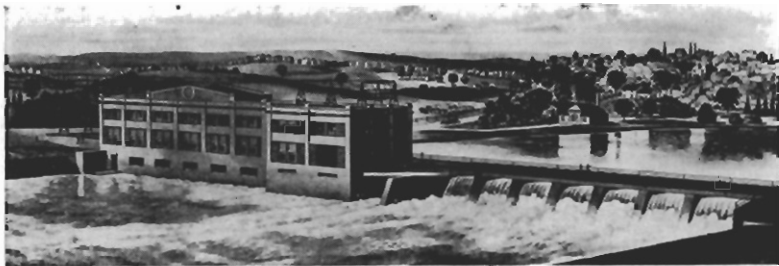
Power House No. 2, Peterboro, Ont.
