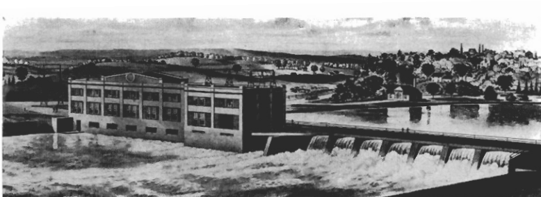
Power House No. 2, Peterboro, Ont.
