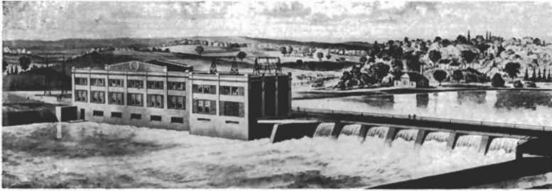
Power House No. 2, Peterboro, Ont.
