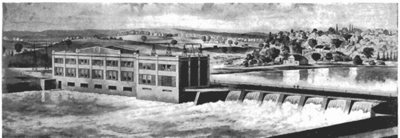
Power House No. 2, Peterboro, Ont.
