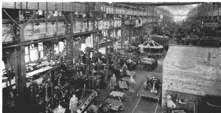
Main Machine Shop, Peterboro Works
