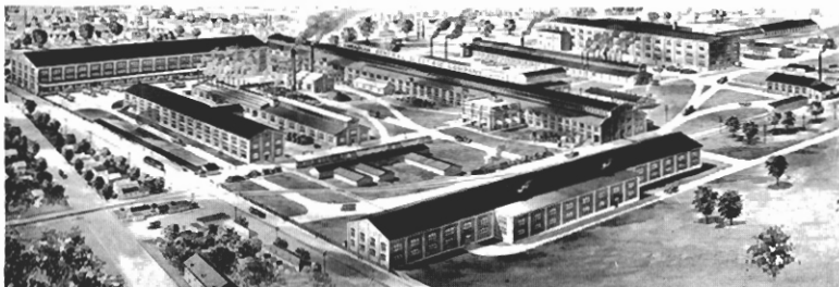
Main Electrical Works, Peterboro, Ont.
