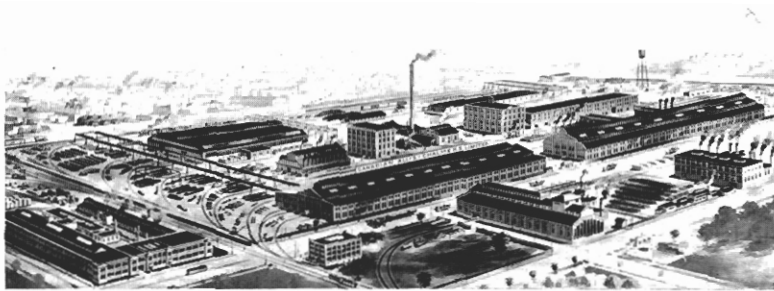
Canadian Allis-Chalmers, Limited, Works, Toronto, Ont.
