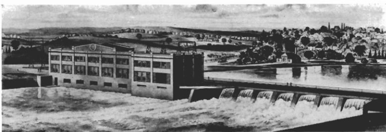
Power House No. 2, Peterboro, Ont.
