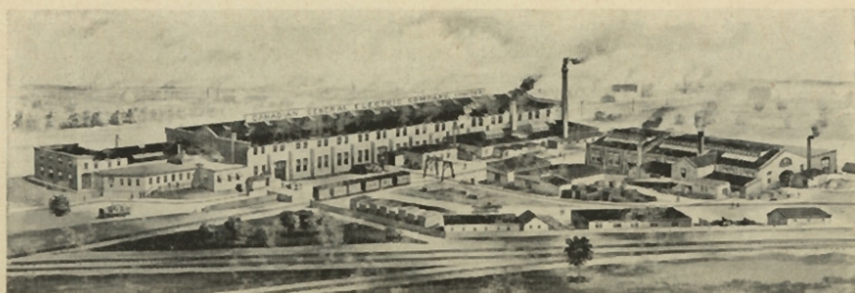
Electrical Supply Works, Toronto, Ont.
