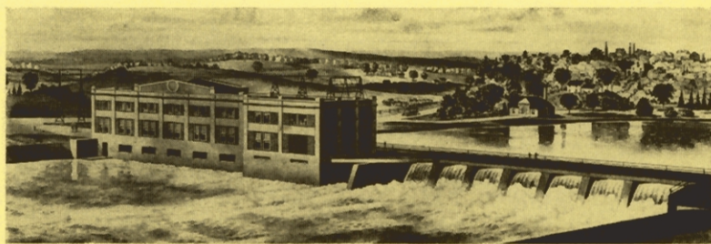
Power House No. 2, Peterboro, Ont.
