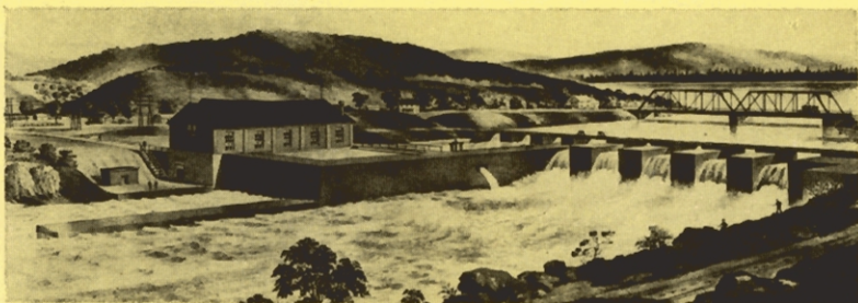
Power House No. 1, Peterboro, Ont.
