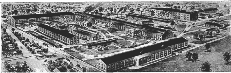
Main Electrical Works, Peterboro, Ont.
