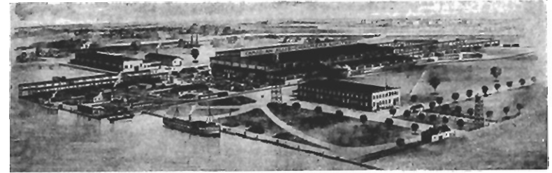
Bridge Works, Bridgeburg, Ont.
