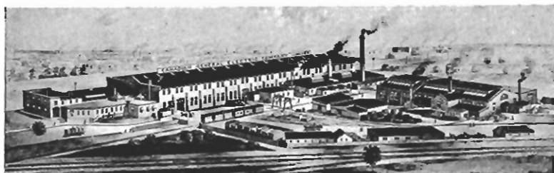
Electrical Supply Works, Toronto, Ont.
