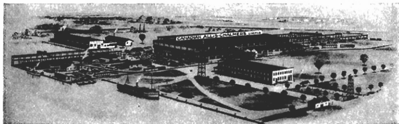
Bridge Works, Bridgeburg, Ont.
