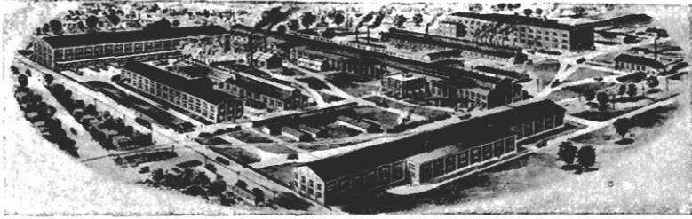
Main Electrical Works, Peterboro, Ont.
