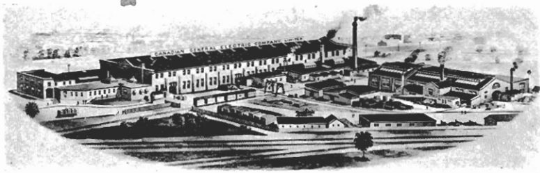
ELECTRICAL SUPPLY WORKS, TORONTO, ONT.
