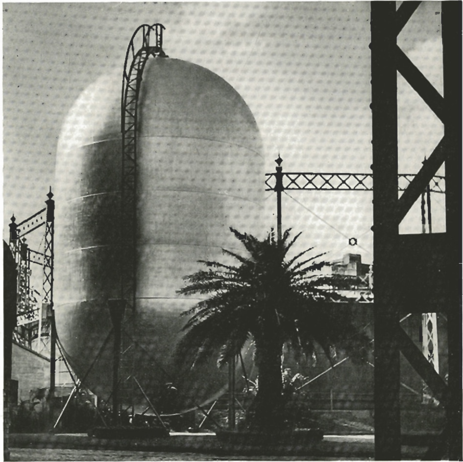
TYPICAL HIGH PRESSURE GAS HOLDER, 3000 CUBIC METRE CAPACITY, SÃO PAULO
