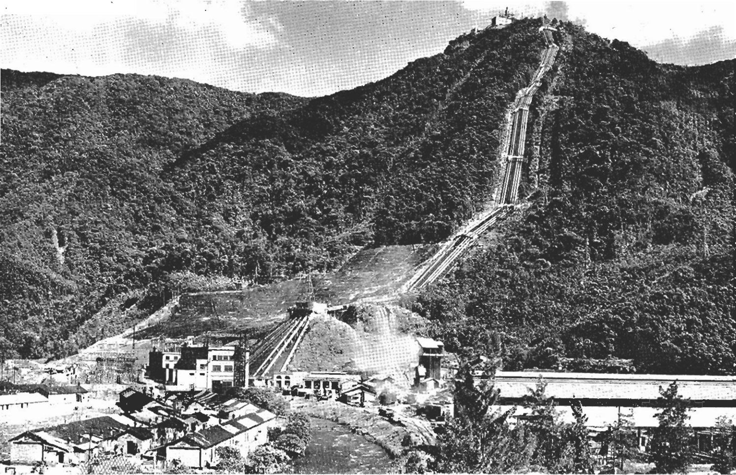
SERRA DO CUBATÃO GENERATING STATION, INSTALLED CAPACITY 407,847 KW, OPERATING UNDER 2358 FT. HEAD.
