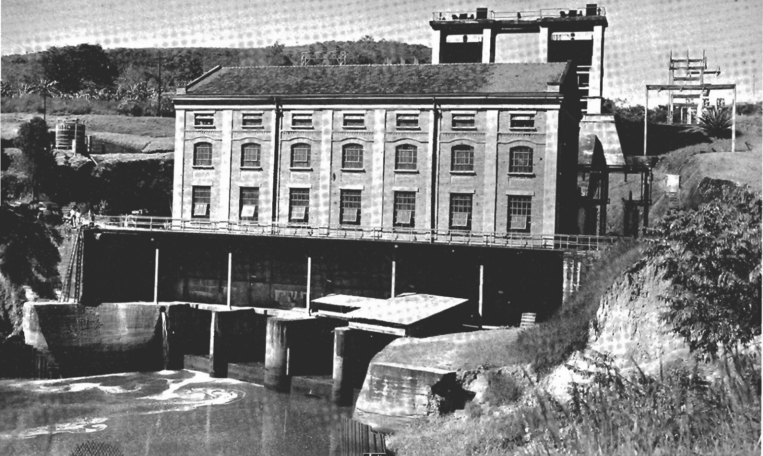
RASGÃO GENERATING STATION ON THE TIETÉ RIVER, STATE OF SÃO PAULO, WITH AN INSTALLED CAPACITY OF 18,539 KW
