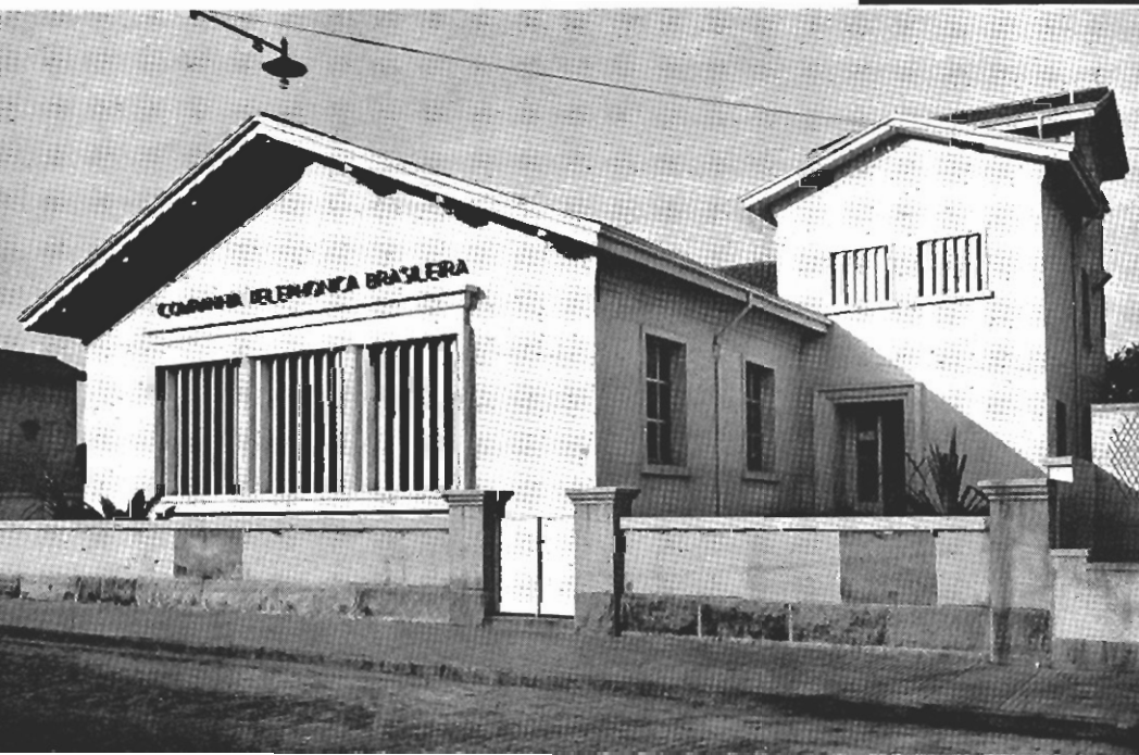
NEW SANTOS AUTOMATIC TELEPHONE OFFICE IN RESIDENTIAL DISTRICT
