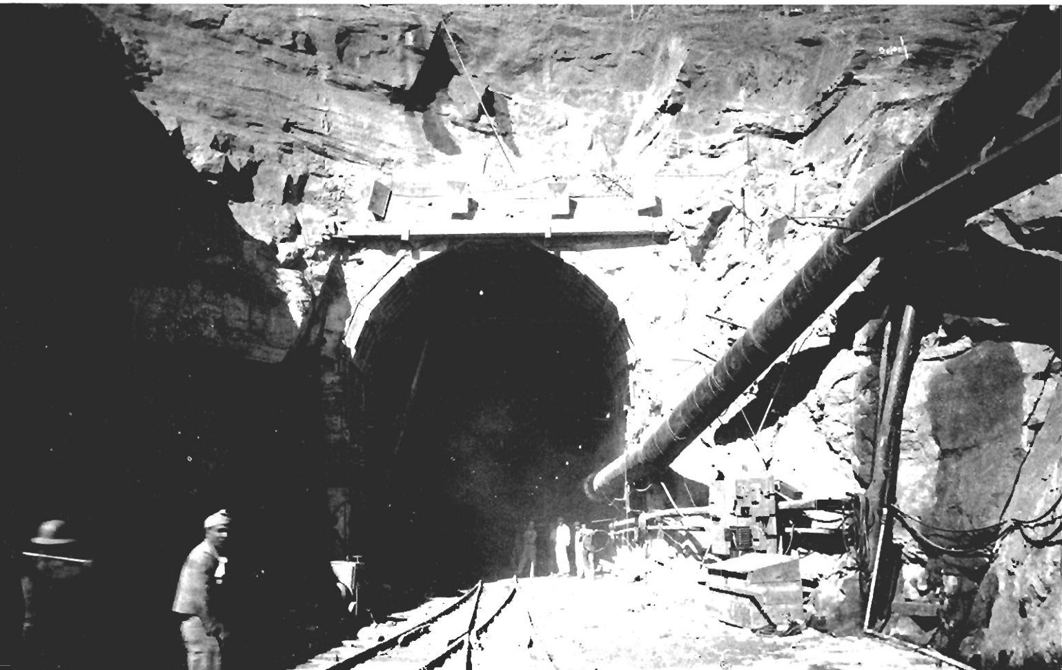
SANTA CECILIA TUNNEL ENTRANCE
