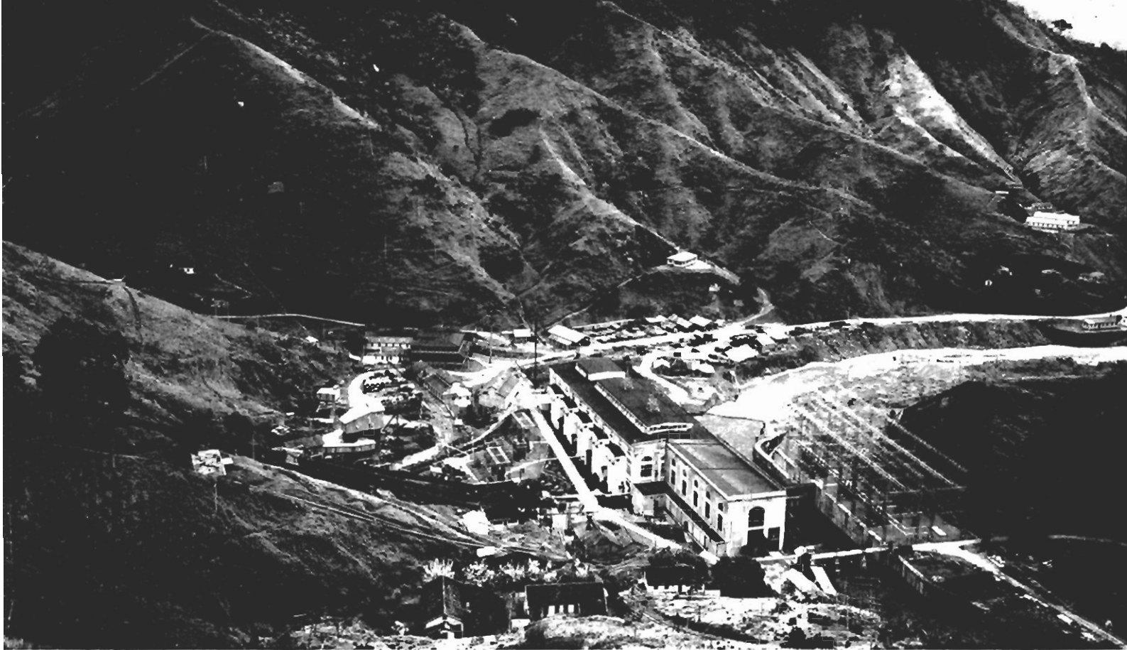
FONTES POWERHOUSE SHOWING EXTENSION FOR THE NEW UNITS
