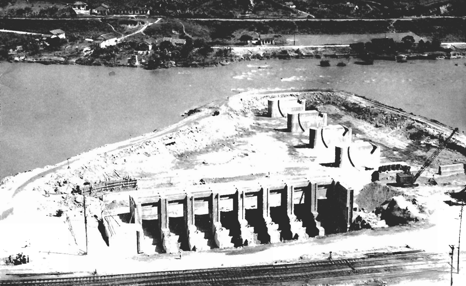
SANTA CECILIA DAM PIERS AND PUMP HOUSE FOUNDATIONS
