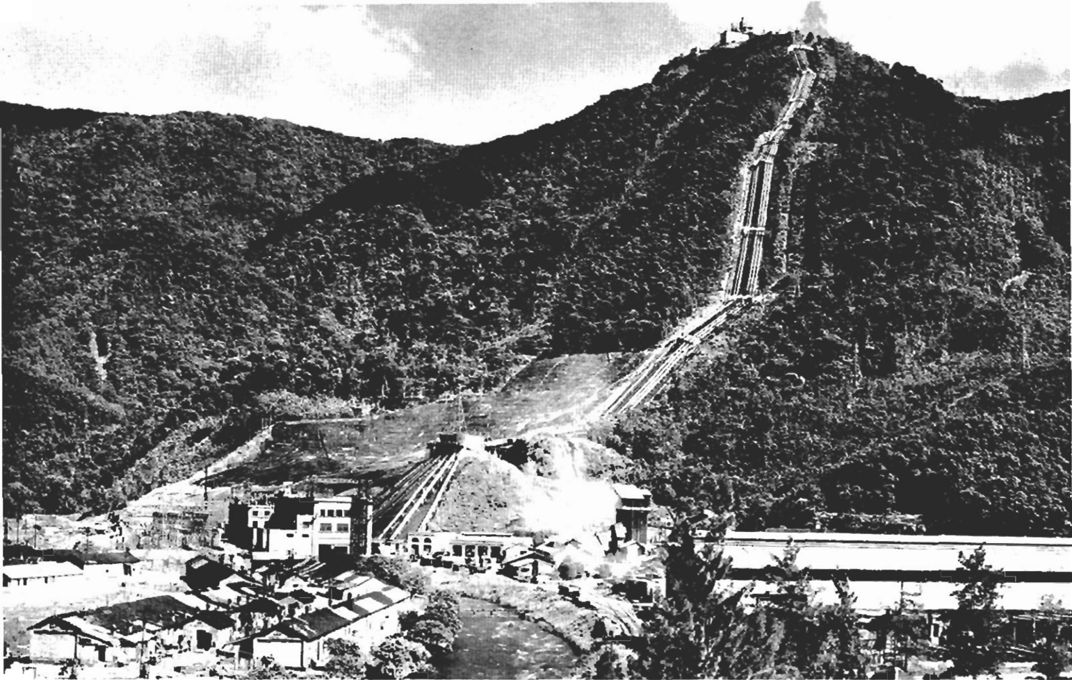
SERRA DO CUBATÃO HYDRO-ELECTRIC PLANT SHOWING POWERHOUSE, PENSTOCKS AND SURGE TANK (STATIC HEAD 2358 FT.)
