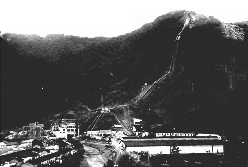
Serra da Cabanão Hydro electric Plant showing Penstocks and Powerhouse - Static Head 1,118 feet alt. near
