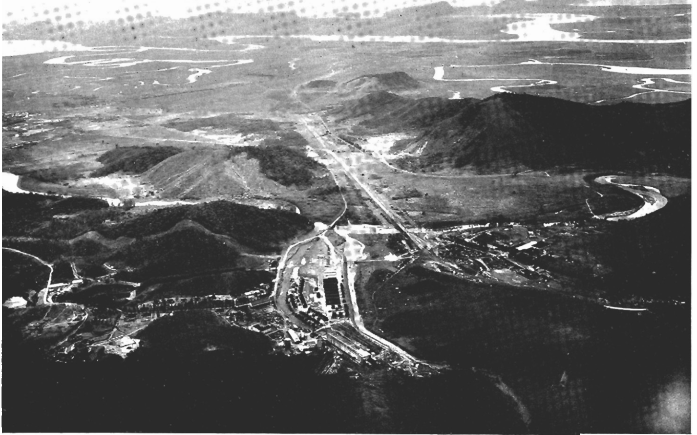
View taken from the top of the Serra plateau looking towards the ocean and showing the Cubatão Powerhouse 2,400 feet below.
