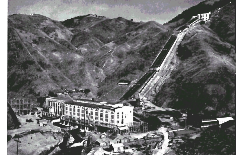
Ribeirão das Lage Hydro electric Plant showing Valanches, Penstocks and Powerhouse - Static Head 1,118 feet alt. near
