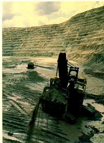
Big bite is taken by 22-yard shovel in the Lornex pit. Haulage volume will increase to 95 million tons of ore and overburden per year as a result of current expansion.
