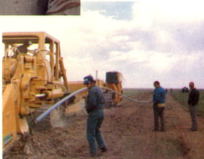
South Eastern 'ploughing-in' a steel gas-gathering line in southern Alberta.
