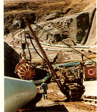
O.J. PIPELINES LAID THE FIRST X80 PIPE IN CANADA FOR NOVA CORPORATION IN THE DRUMHELLER AREA OF ALBERTA.
