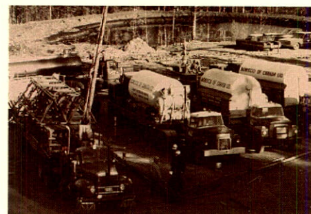
An atomized acid job in progress May, 1967.
