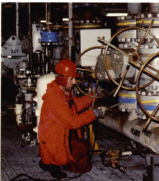
Probing for leaks on valve flanges.
