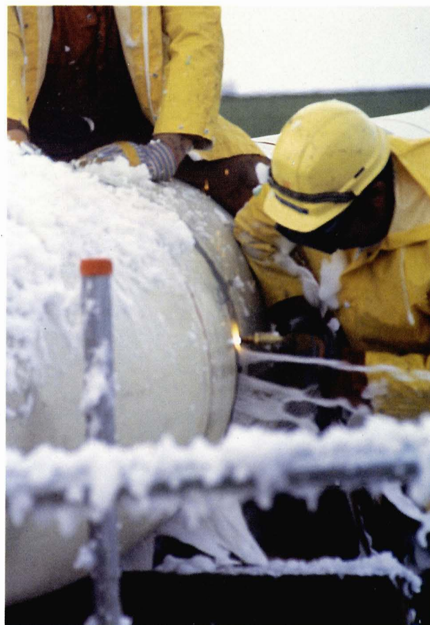
Nitrogen Foam Inerting "Hot Cut".
