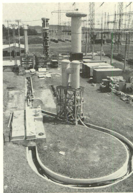
INSTALLING AN OIL-INSULATED AC 800-KV CABLE IN A DUCT AT THE UNDERGROUND CABLE TESTING FACILITY (HIGH-VOLTAGE LABORATORY; CABLES AND INSULATION, IREQ).
