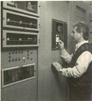
Roger Jutras tests the operating characteristics of one of the load behavior measurement systems installed in Hydro-Québec substations.
