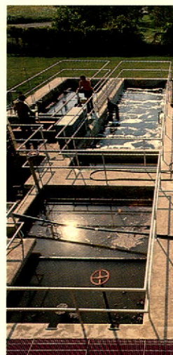
Waste Water Treatment
