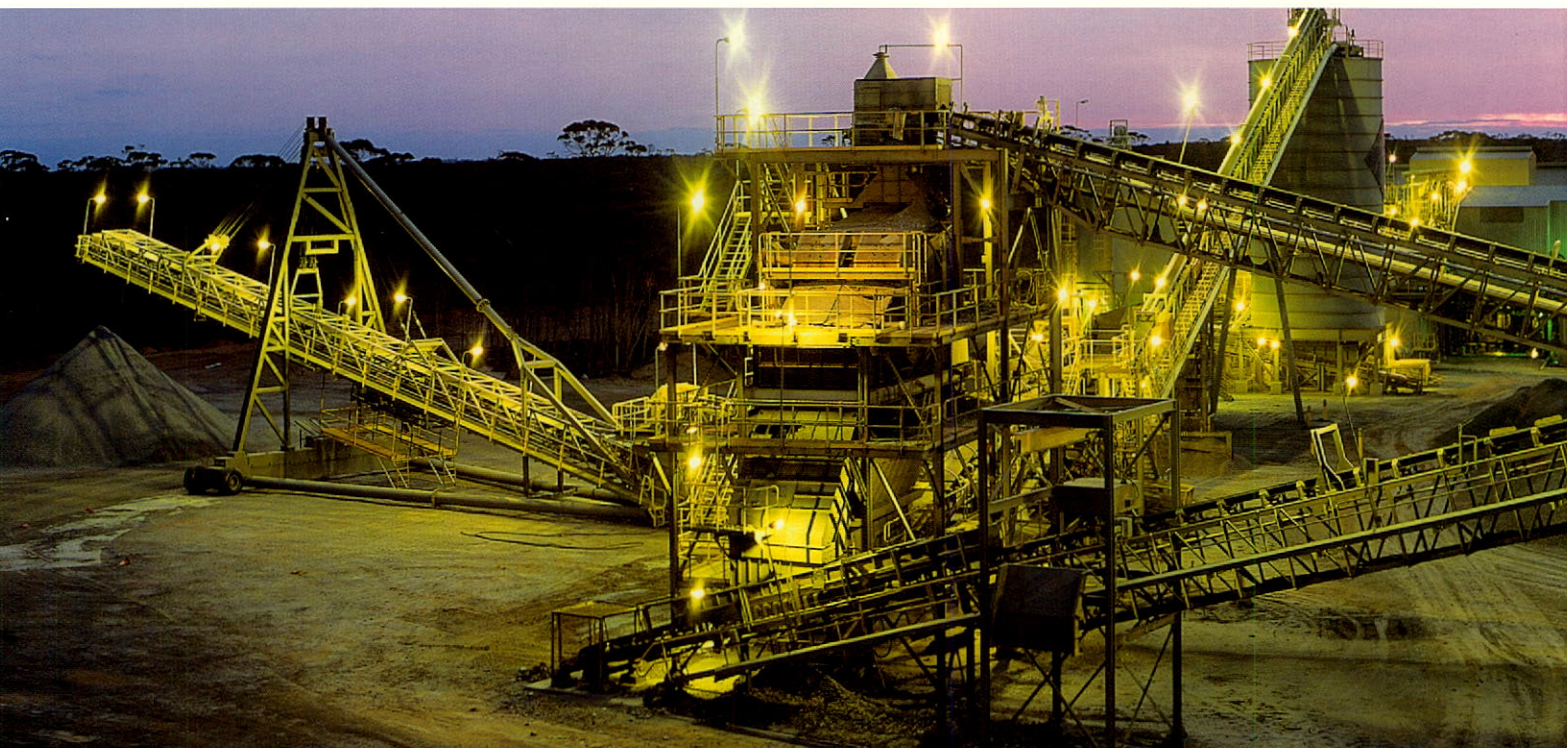
Process Plant at Lake Johnston
