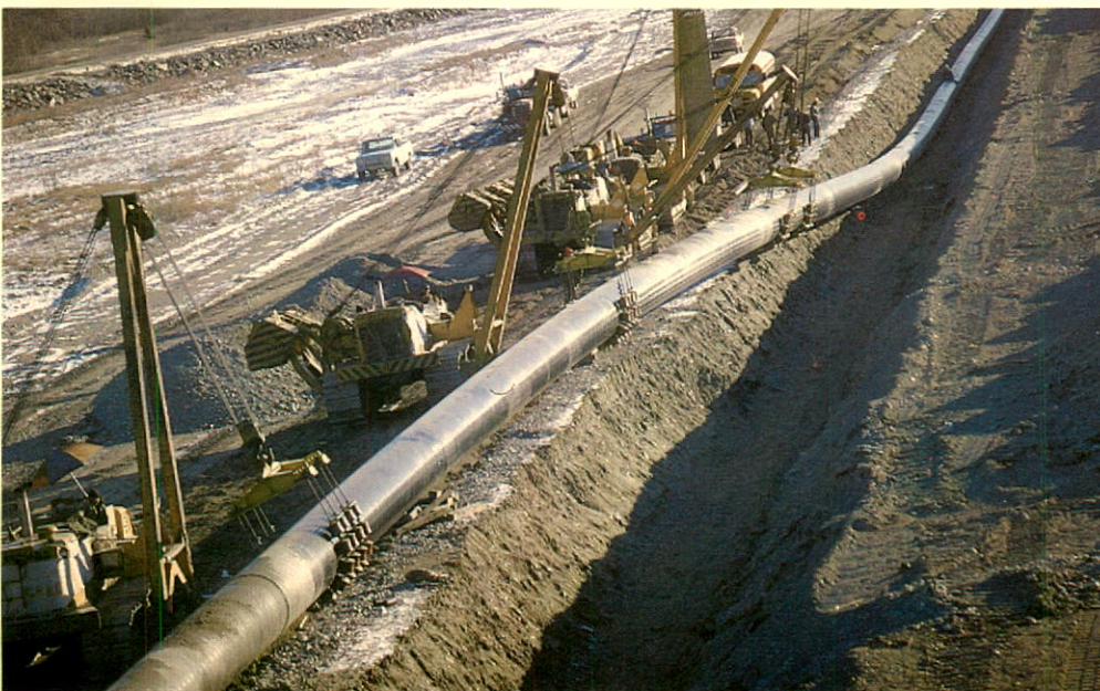
Lowering in of 48" oil line into ditch.
