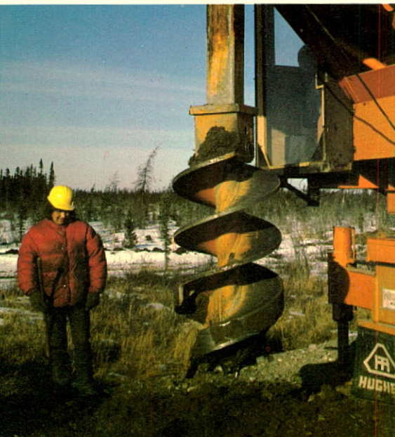
Drilling one of the many thousands of holes required for the vertical support members to support the above ground pipe.
