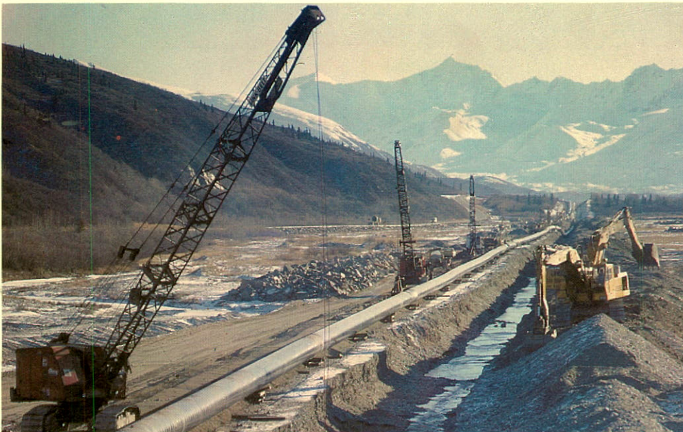
Clamming the ditch prior to lowering in of pipe.
