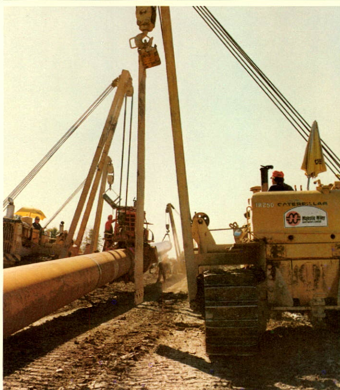
A portion of the company crews constructing a 42" gas line project in Southern Ontario during 1975. The crews shown are the pipe gang, the tape crew and the tie in crew.
