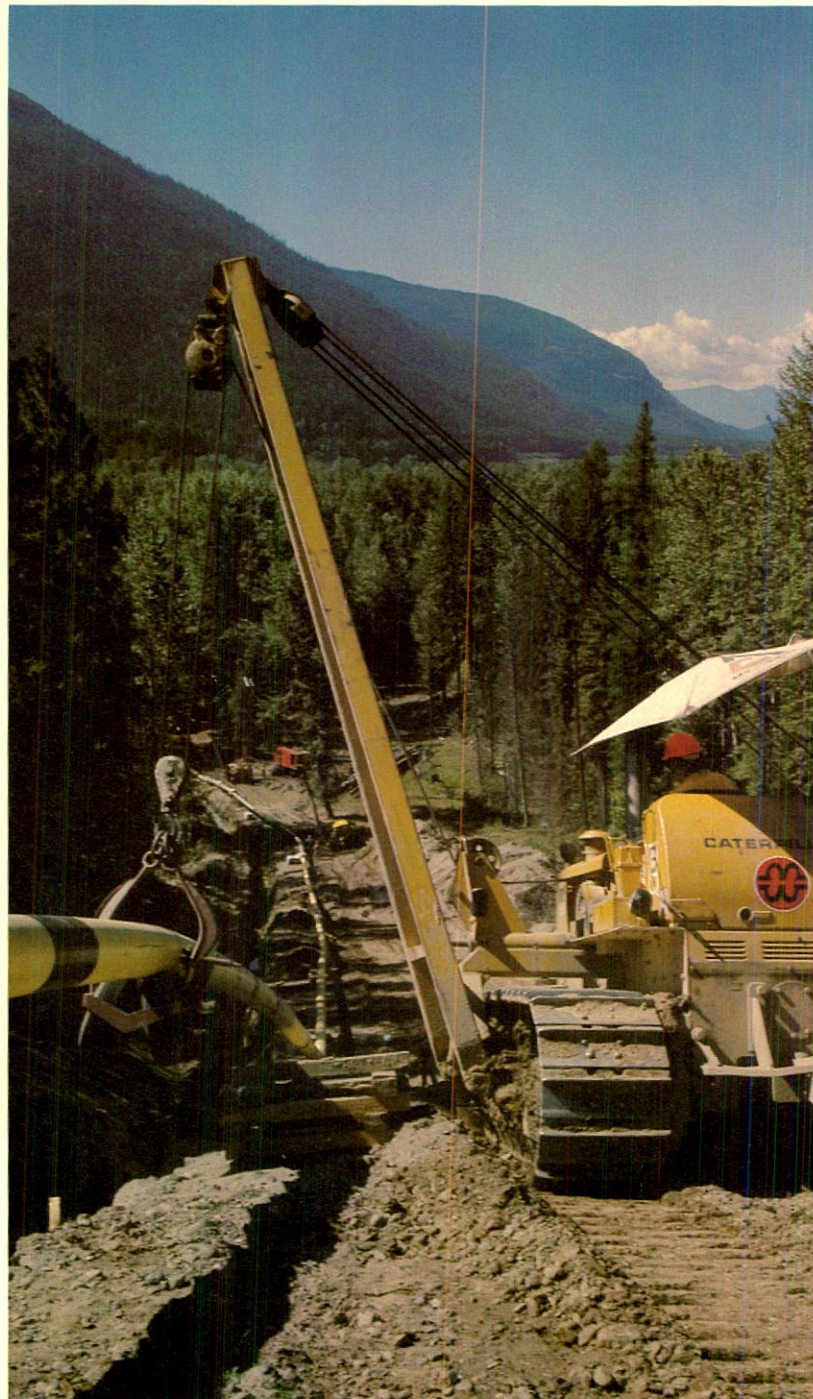
Lowering the pipe into the ditch.
