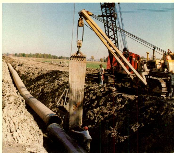
A portion of the company crews constructing a 42" gas line project in Southern Ontario during 1975. The crews shown are the pipe gang, the tape crew and the tie in crew.
