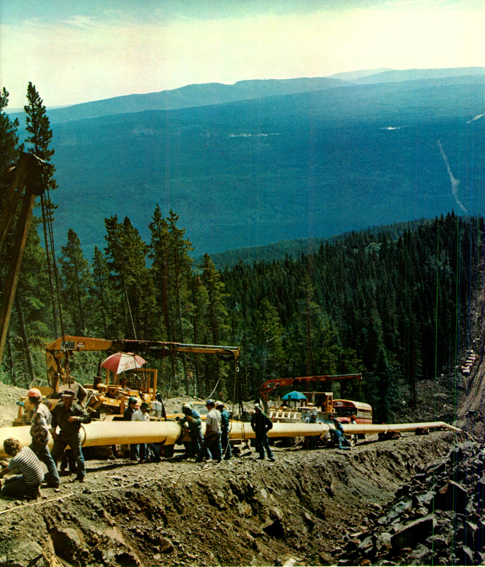
A stringer bead and hot pass welding crew working on the Grizzly project. Following this operation, a filler and capping welding crew will complete the welding process.
