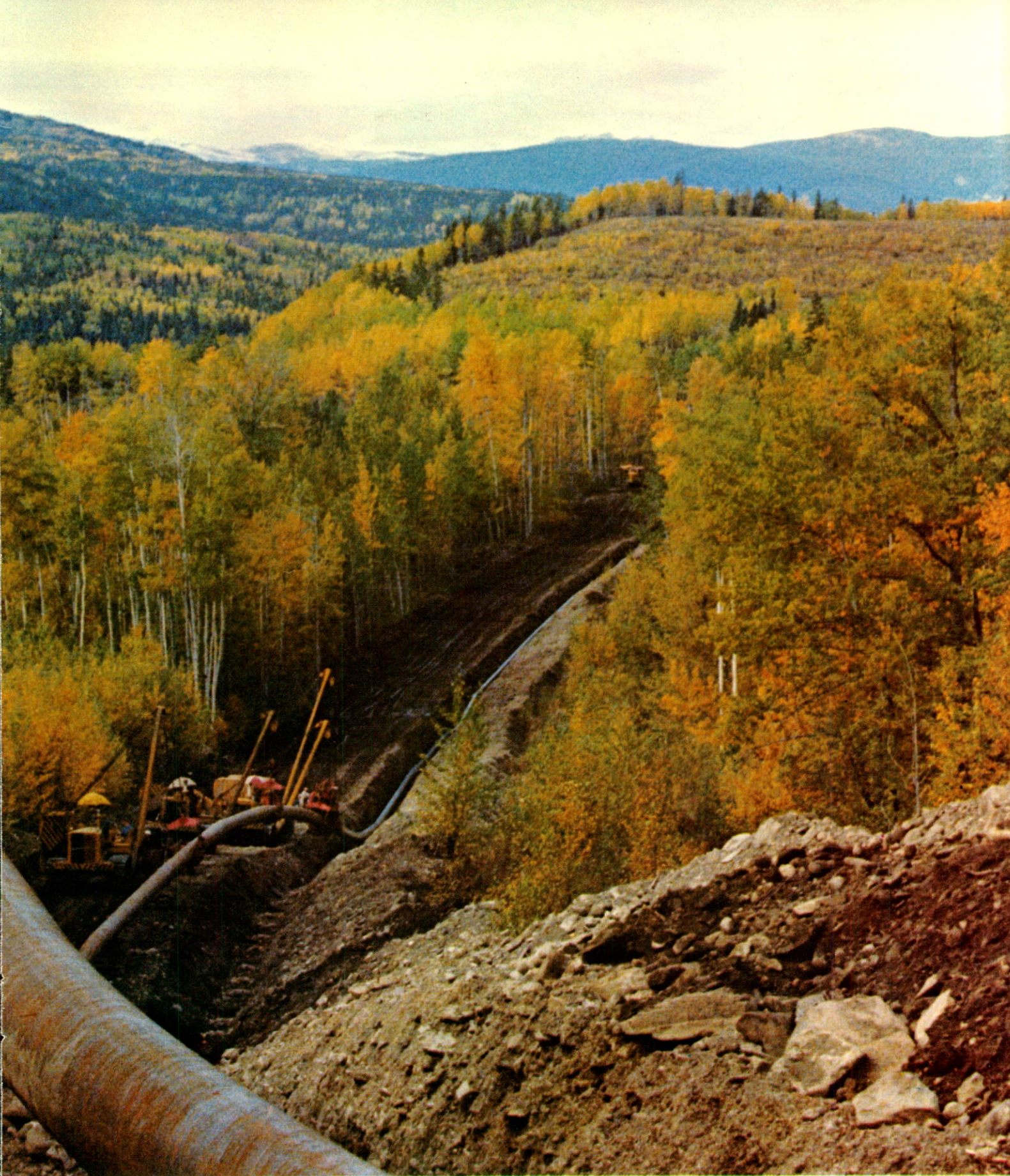
Company crew taping and lowering in 91.44 cm. (36") pipe for project in northwestern British Columbia.
