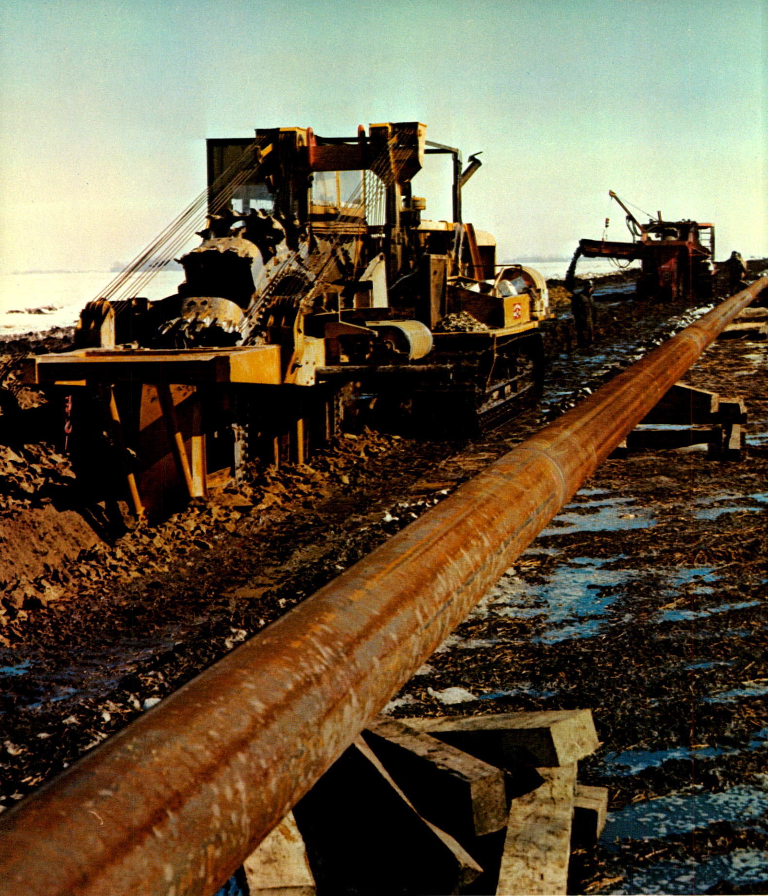
Pipeline trenching operation for winter construction in North Dakota. The first ditching machine is removing the topsoil, which will be replaced on the right of way after the pipeline has been buried.
