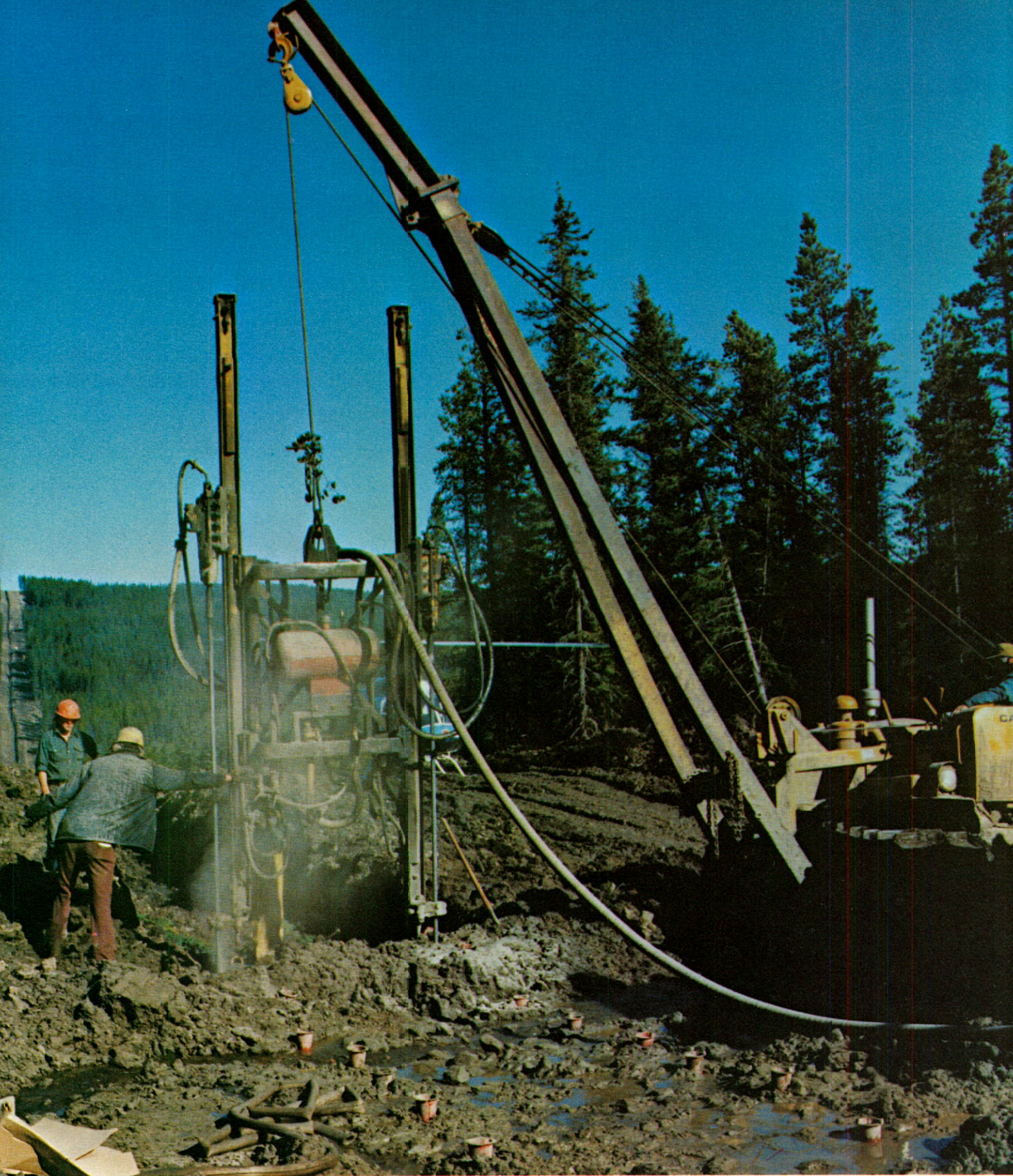
Company crew operating a twin drill on the Grizzly project prior to the removal of ditch rock by blasting.
