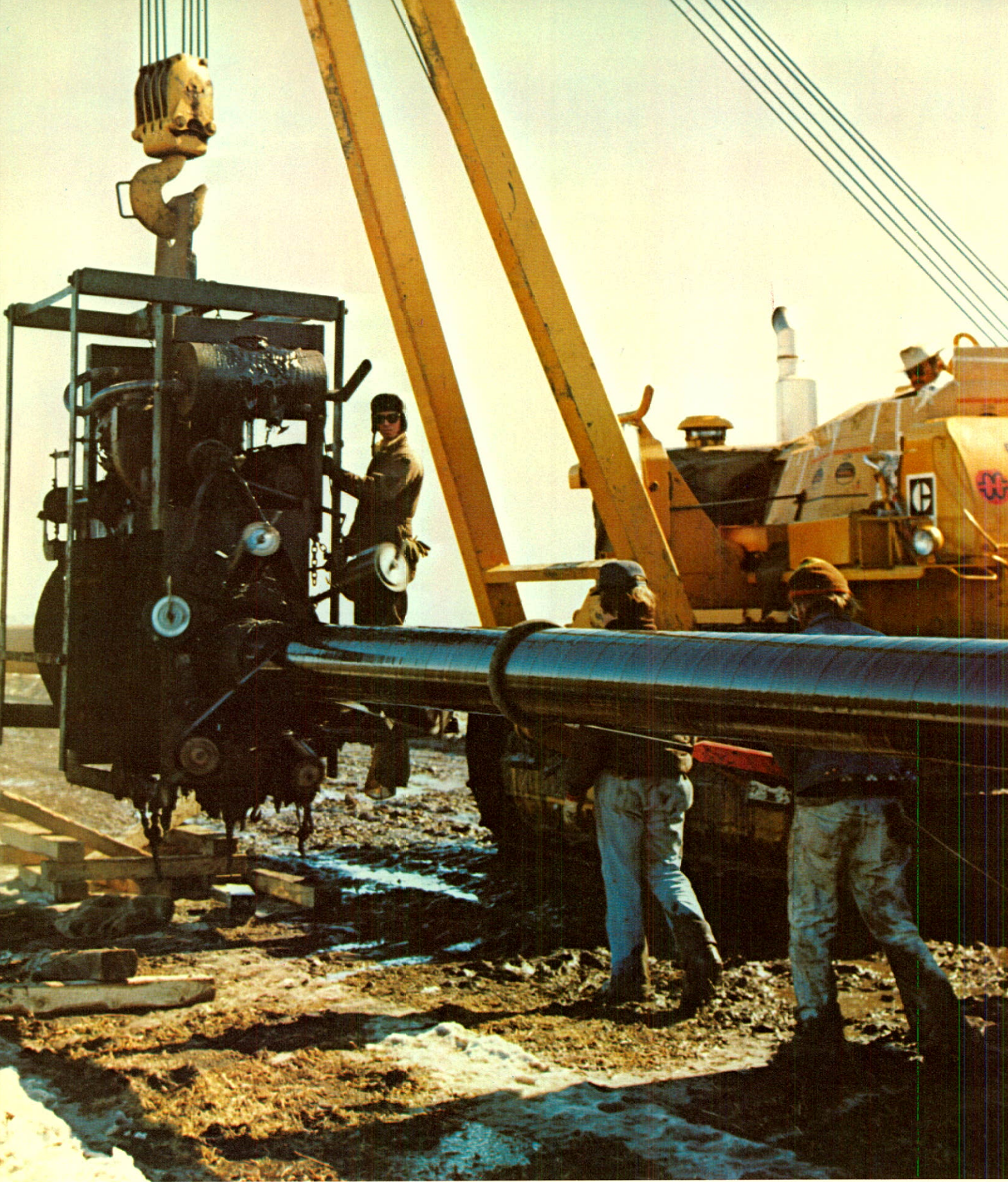
A line-travel clean, prime and tape machine used to prepare the pipe prior to burial.
