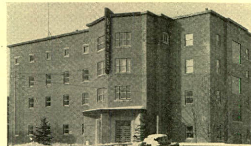
COMMUNITY CENTER BUILDING, Rimouski, P.Q.
