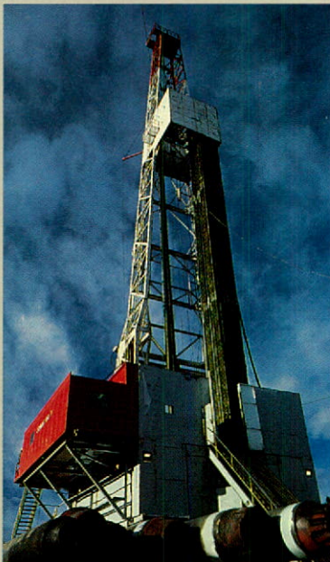
A drilling rig operating in southern Saskatchewan
