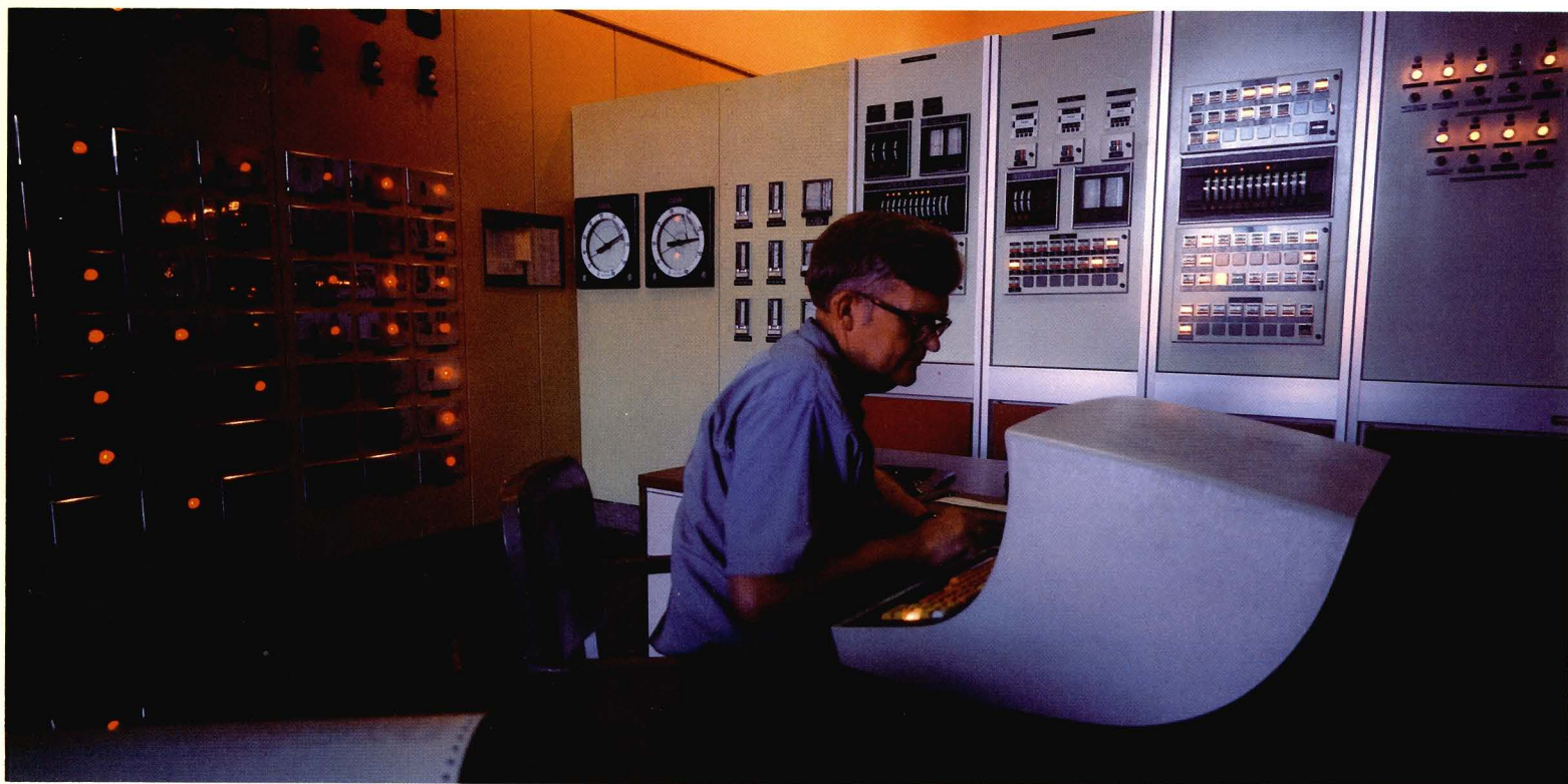
Lawrenceburg computer is only one in the industry for controlling distillery processes.
