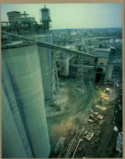
General Portland's Whitehall Cement Plant in Pennsylvania employs the cost-efficient pre-heater technology, which reduces kiln operating costs.
