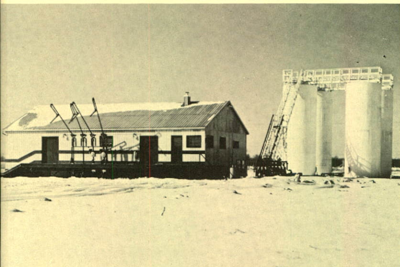
Typical Bulk Plant
