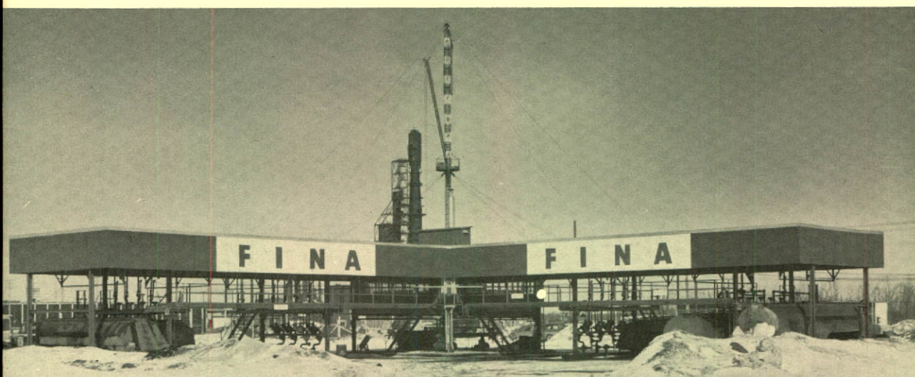
Modern Tank Wagon Loading Rack, Montreal Bulk Plant
