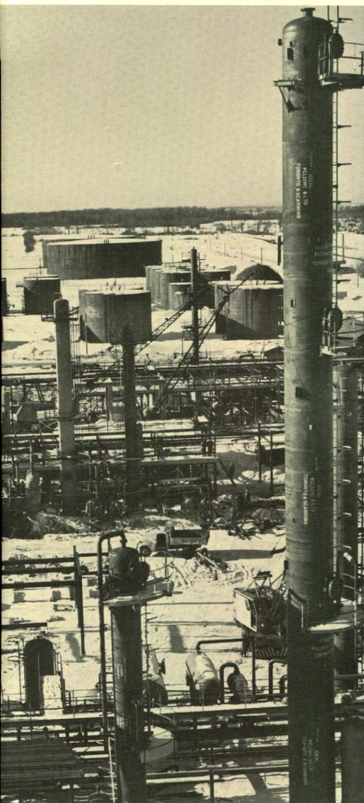
Construction activity — Montreal Refinery
