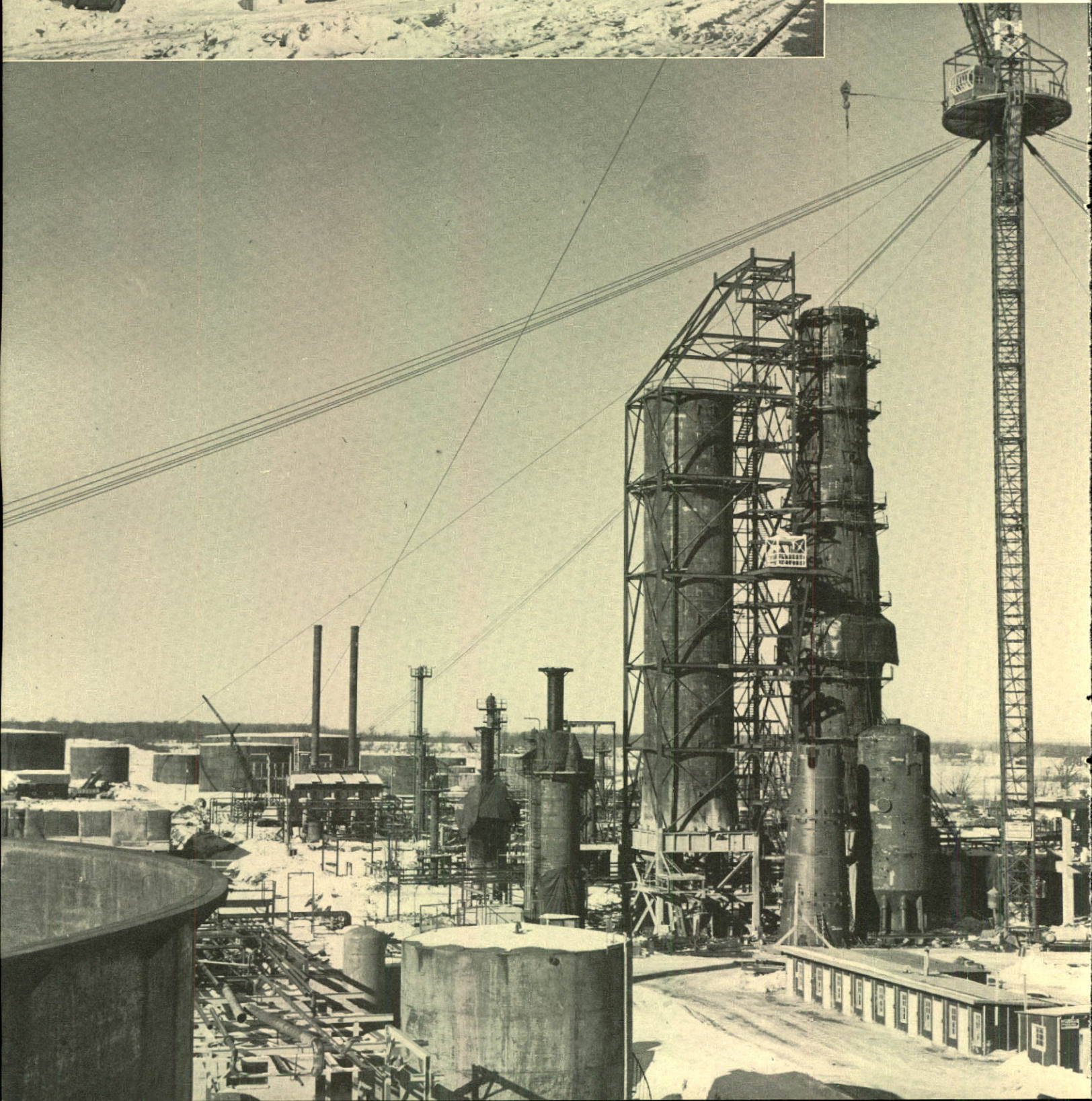
Catalytic Cracking Tower being erected
