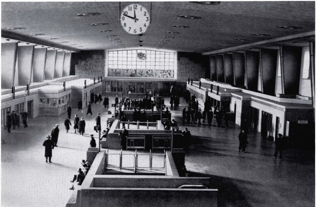
This view shows approximately one-half of the concourse. The entrance to the restaurant is seen in the background of the photograph; down the centre are the stairways and escalators joining the concourse and the train platforms.
