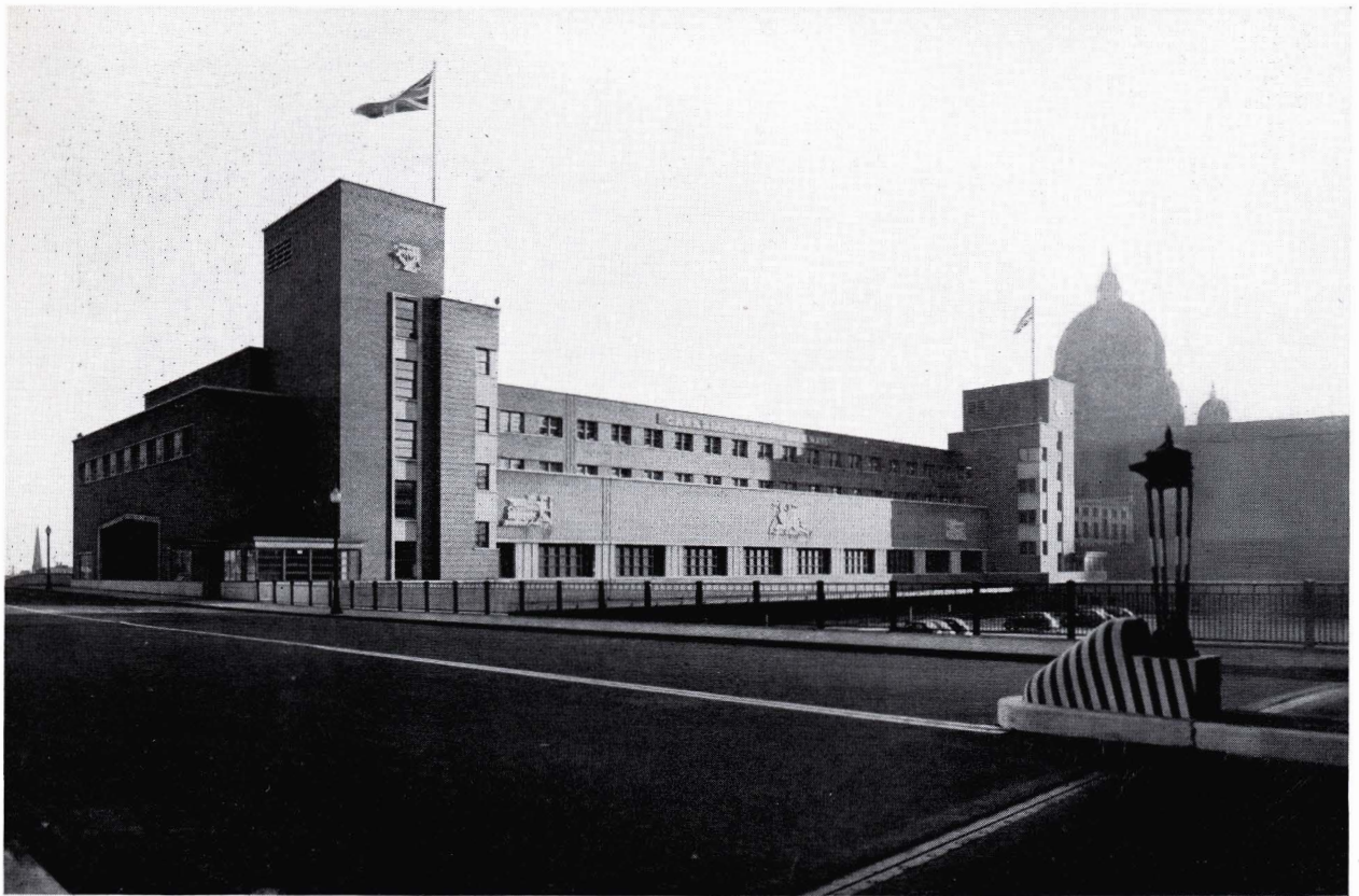
The north and east façades of the station building.
