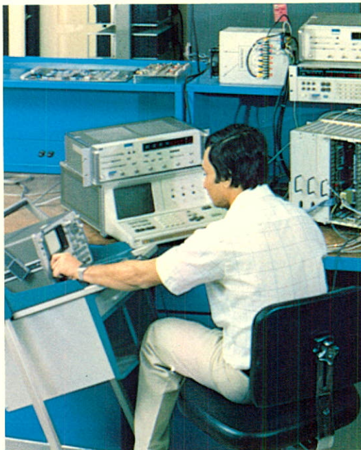
Time Division Multiple Access/Digital Speech Interpolation (TDMA/DSI) equipment enhances the capacity of satellite communications systems.
