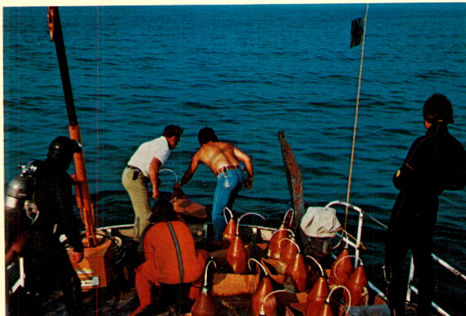
The crew aboard the diving boat David Allen on Lake Erie is placing specially designed explosive charges on the lake bottom for the excavation of a pipeline trench in rock.
