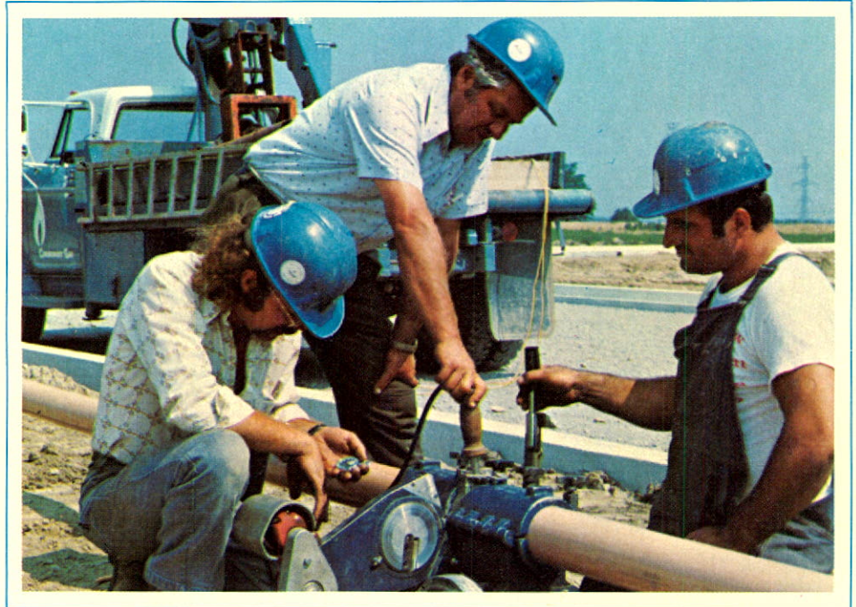
(Left to right) Wilf MacDonald, Gino Panetta (construction foreman) and C. Girdali heat fusing a plastic gas main being installed to serve an industrial complex in Scarborough.
