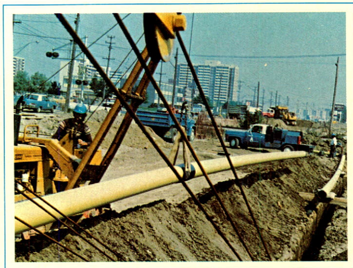
One of Consumers' construction crews relays an 8" steel main necessitated by the building of a railway underpass in Scarborough. In projects of this kind, Consumers' works closely with other utilities and the municipal departments involved.
