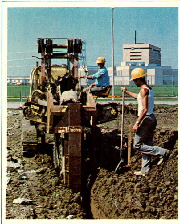
Adrian Snoeys and Vitto Vidiri operate trenching equipment for Cliffside Pipelayers Limited, one of the contractors employed by Consumers' Gas, to lay mains to extend service to new sub-divisions. Contractors supplement Consumers' own work crews to equalize work loads and meet the fluctuating demands created by the seasonal nature of our business.
