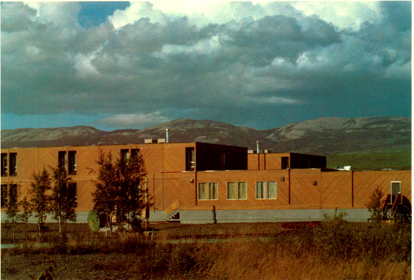
Imperial Oil's permanent base camp at Norman Wells, N.W.T., built in 1980 by Custom Structures
