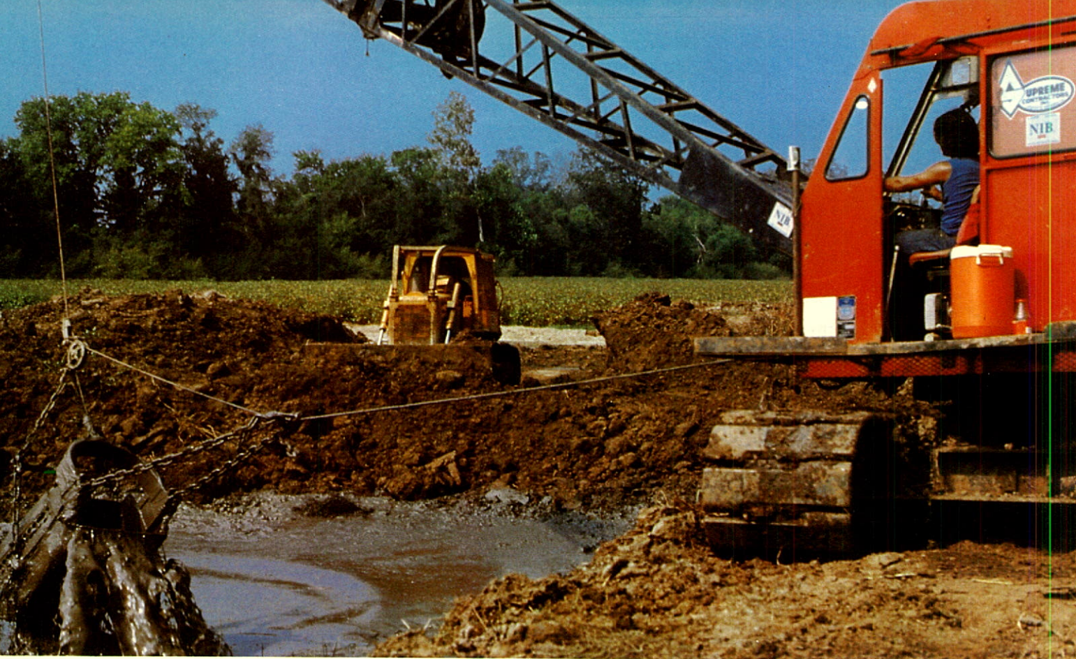
A Supreme Contractors, Inc. dragline cleaning up a drill site near False River, Louisiana
