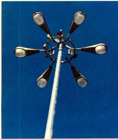
Polesystems developed a new high mast raising and lowering device with a patented latching device.
