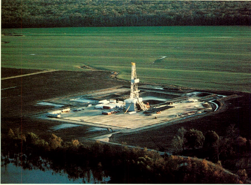
Supreme Contractors, Inc. completed a 6-acre hardwood board drill site.
