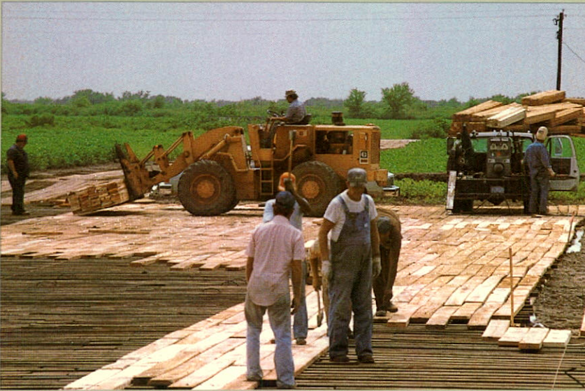
Supreme Contractors, Inc. builds hardwood board roads and drill sites and does production equipment installation and maintenance.
