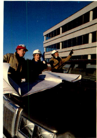
GE Canada's flagship head office, now under construction in Mississauga, Ontario, will be completed in the Fall of 1987.
