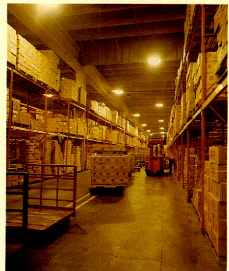
New Lumaglow® fixtures installed in Dominion Store warehouse.
