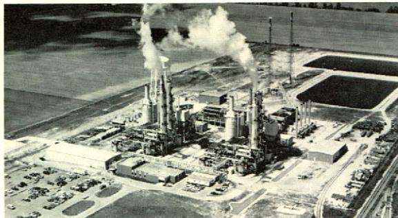
Petroleum liquids imported from Canada are converted to synthetic natural gas at Columbia's plant in Green Springs, Ohio. SNG plant provided 6% of total System supply in 1979.
