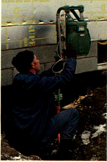
Columbia's retail companies set more than 25,700 meters to connect new residential and commercial customers.
