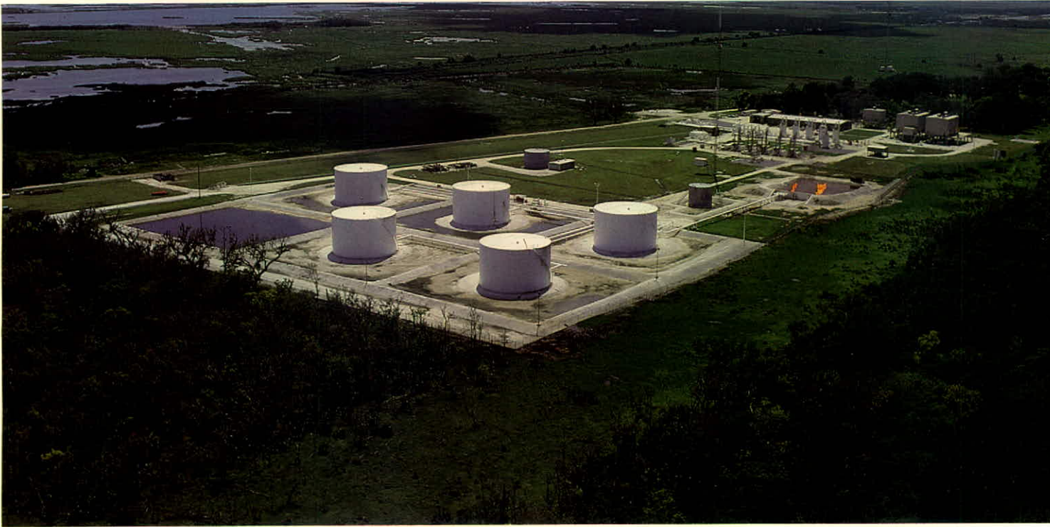
Natural gas from offshore wells passes through this Columbia plant in southern Louisiana for the removal of any liquids or other materials it contains.
