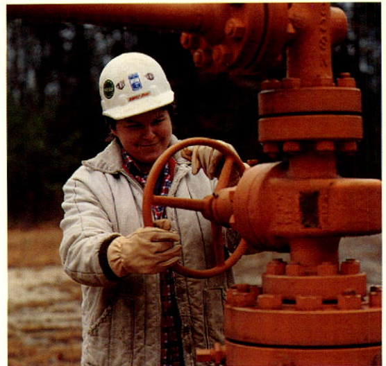
Nancy Kuhl checks a natural gas storage well in West Virginia.
