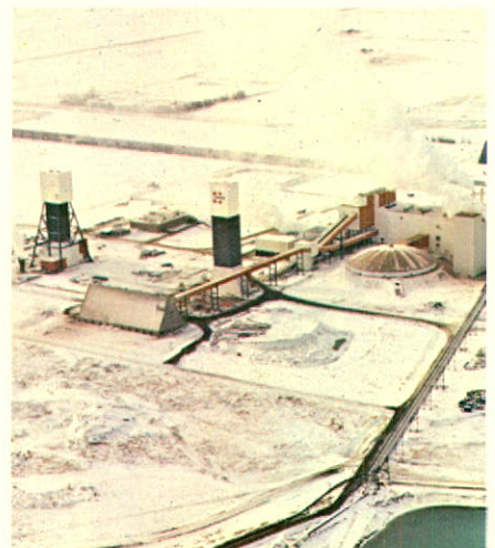
The $31-million expansion program at the Vade Potash Operation was completed in 1982.
